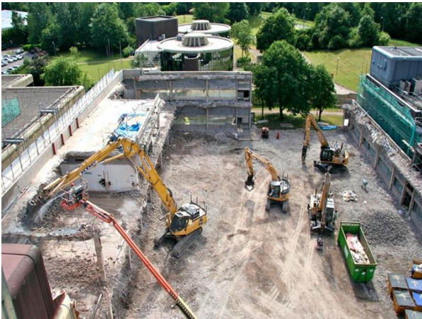
Figure 2: An example of the final stages of decommissioning and clean-up
