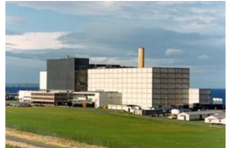
Figure 11: Dounreay PFR when operating.
