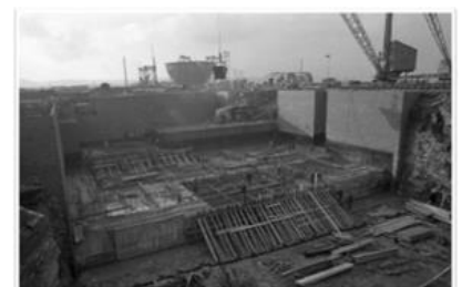
Figure 13: Construction work at Dounreay showing underground structures
